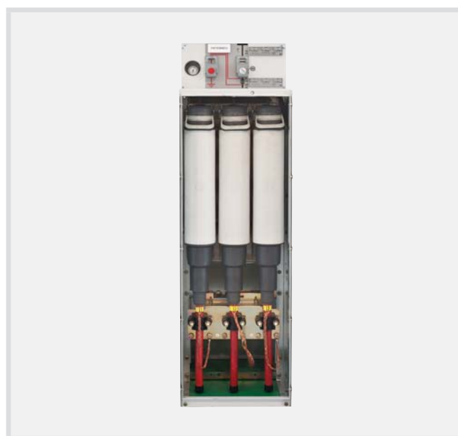
Transformer outgoing panel, front cover opened. With fuse holders and transformer cable sealing end.
