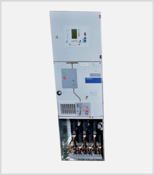
Front view showing open cable termination area with fourfold cable termination
