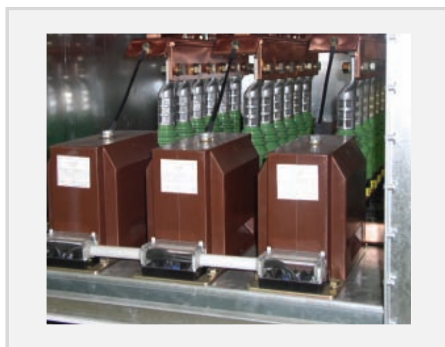
Standard voltage transformers DIN 42600 part 9, front mounted
