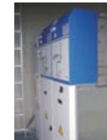
Example: 36 kV OL1L1P configuration inside the wind power generator
